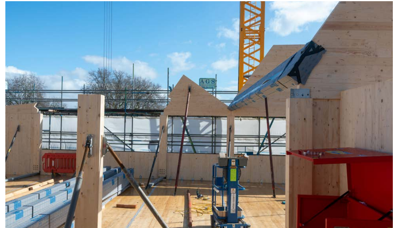
Wood works — BauBuche laminated veneer lumber beams were selected for their strength to carry the sawtooth roof form
