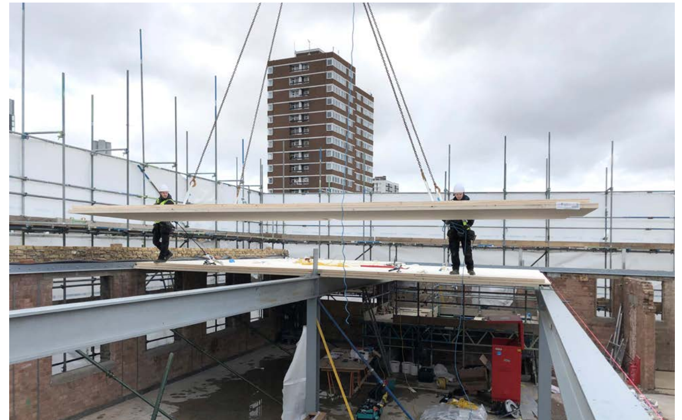
Site savings — using CLT on the new structure and limiting internal finishes reduced on site construction time and embodied carbon
